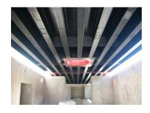
The entire understructure of the scale is undercoated with an asphaltic coating. This significantly increases the scale's life in your environment as compared to others because it drastically reduces the deterioration of the steel.
